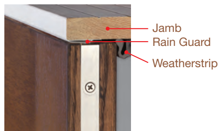
Top of door; exterior view.
